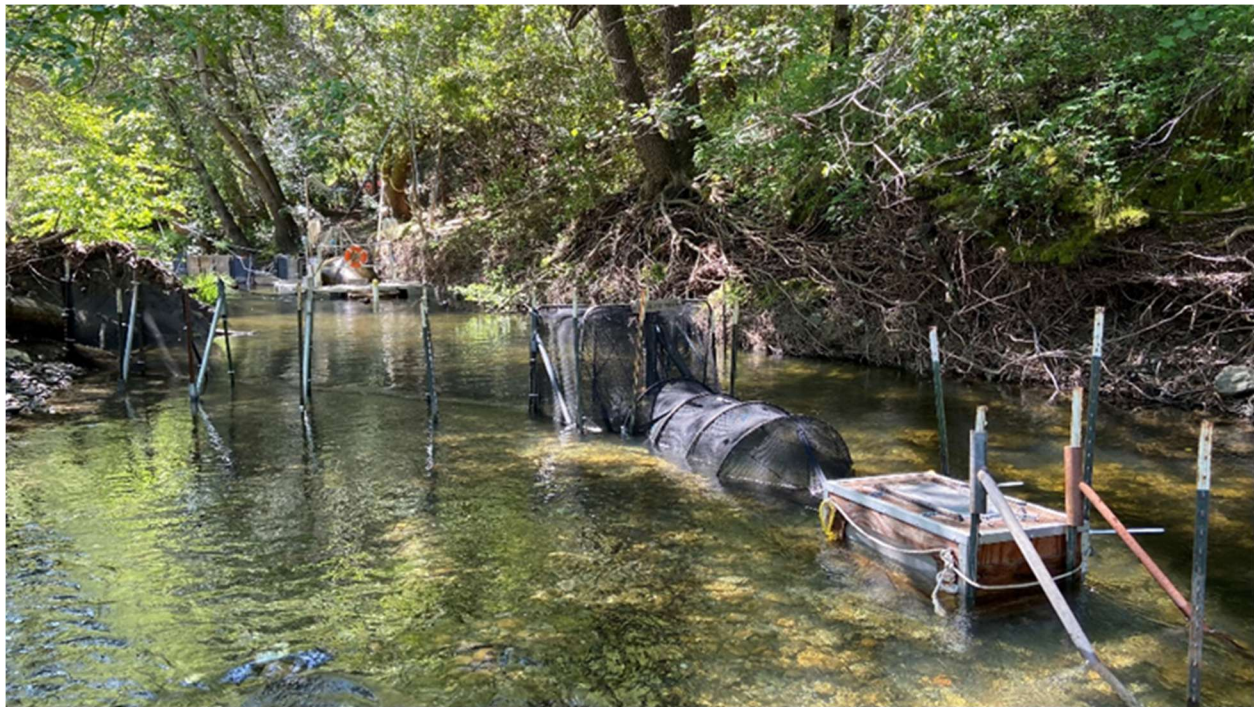
Figure 6-3. Alameda Creek fyke-net trap after installation in April 2024.
